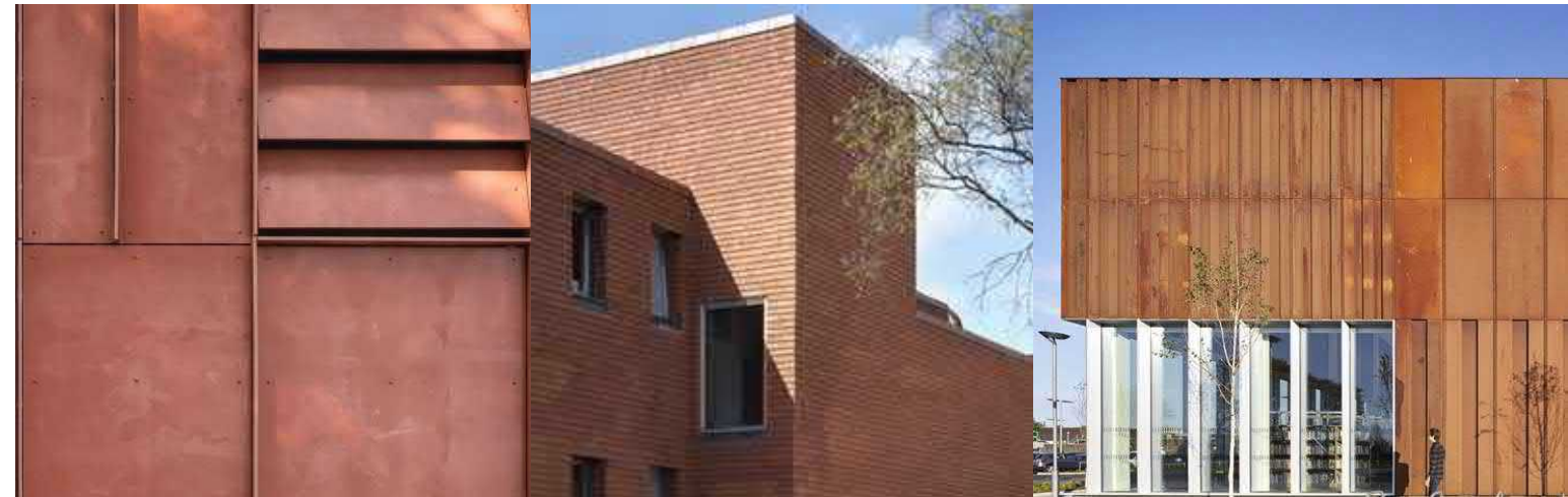
CLADDING MATERIALS WITH 'SOLID' CHARACTER – CEMENTITIOUS PANELS – HUNG TILE – CORTEN/METAL PANELS
